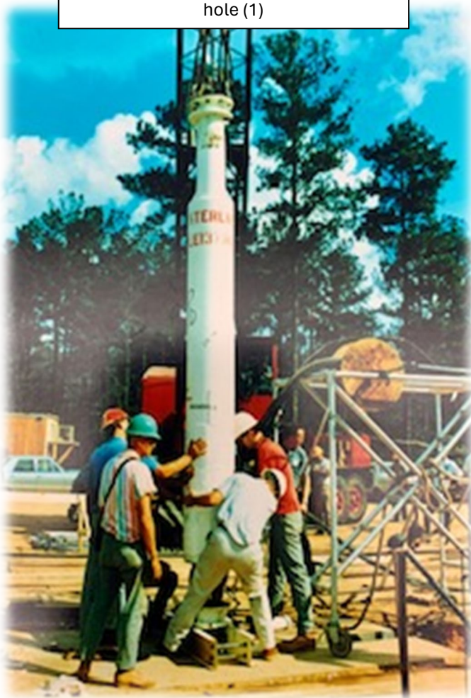
Figure 7. Sterling Package going down hole (1)
