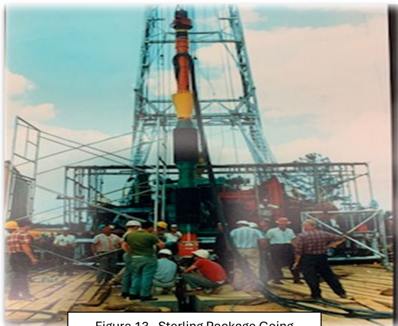
Figure 13. Sterling Package Going Down Hole (2)
